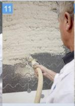
Apply SM700 mortar by hand or machine to a thickness of 5mm
