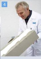
Apply Warm Wall Duo adhesive to the back of the starter panel
