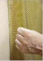
below the surface of lines on the mesh to the mortar and level establish the required 100mm overlap
