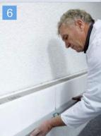
Apply the Quix starter Apply Quix drip bead to a true and straight line line on the lower edge profile to fixed track of the polystyrene board - Alternative method for this is to use a standard Marmorit starter track and fix through to the substrate. Please consult the Marmorit technical department
