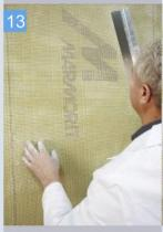
Trowel into the fresh mortar a layer of fabric reinforcing
