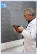
Fix the boards at 4 fixings per sqm for thicknesses up to 60mm. Over 60mm 5 fixings per sqm
